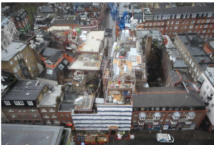
Aerial view of the site
