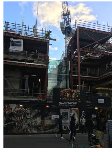
Glass Bridge installation
