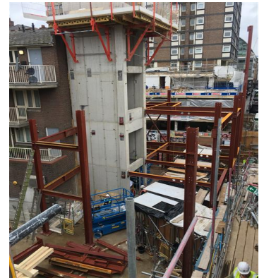
West elevation steel frame
